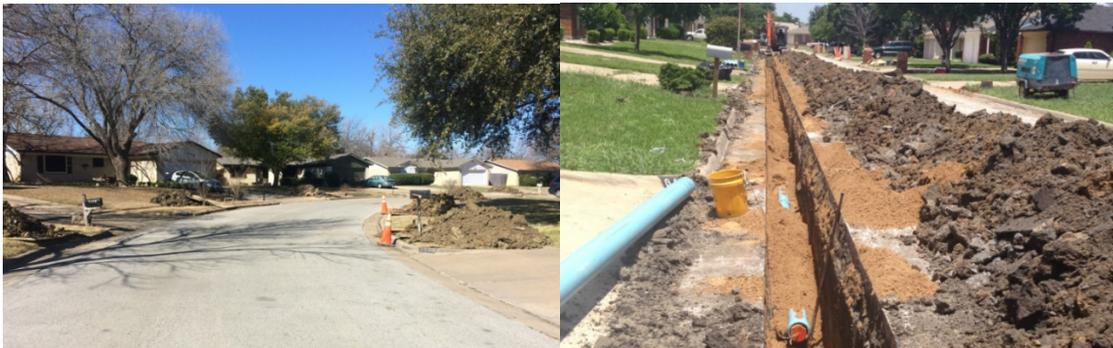
The pre-chlorinated pipe bursting method means the City of Arlington doesn't have to dig an open trench down a street to replace an old water main. That's because 85 percent of the work is done underground.
